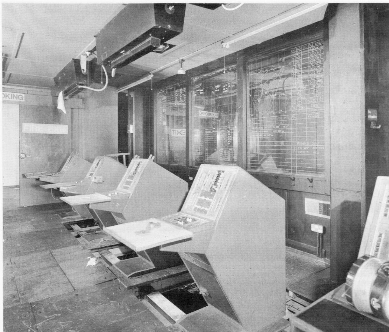
The control cabin built within the receiver hall on the upper floor of the R12. The 'Wendy Cabin', as it became know, was built in 1974/5 following the closure of RAF Patrington allowing Staxton Wold to take full operational control of its own radar picture. Photo by Nick Catford
